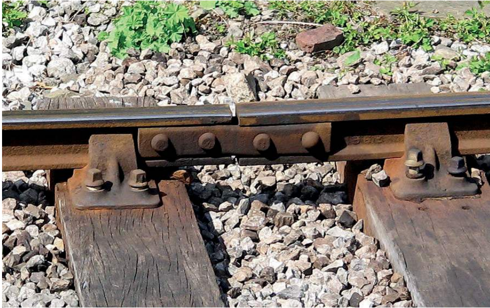
Figure 6: The gaps along railway tracks
